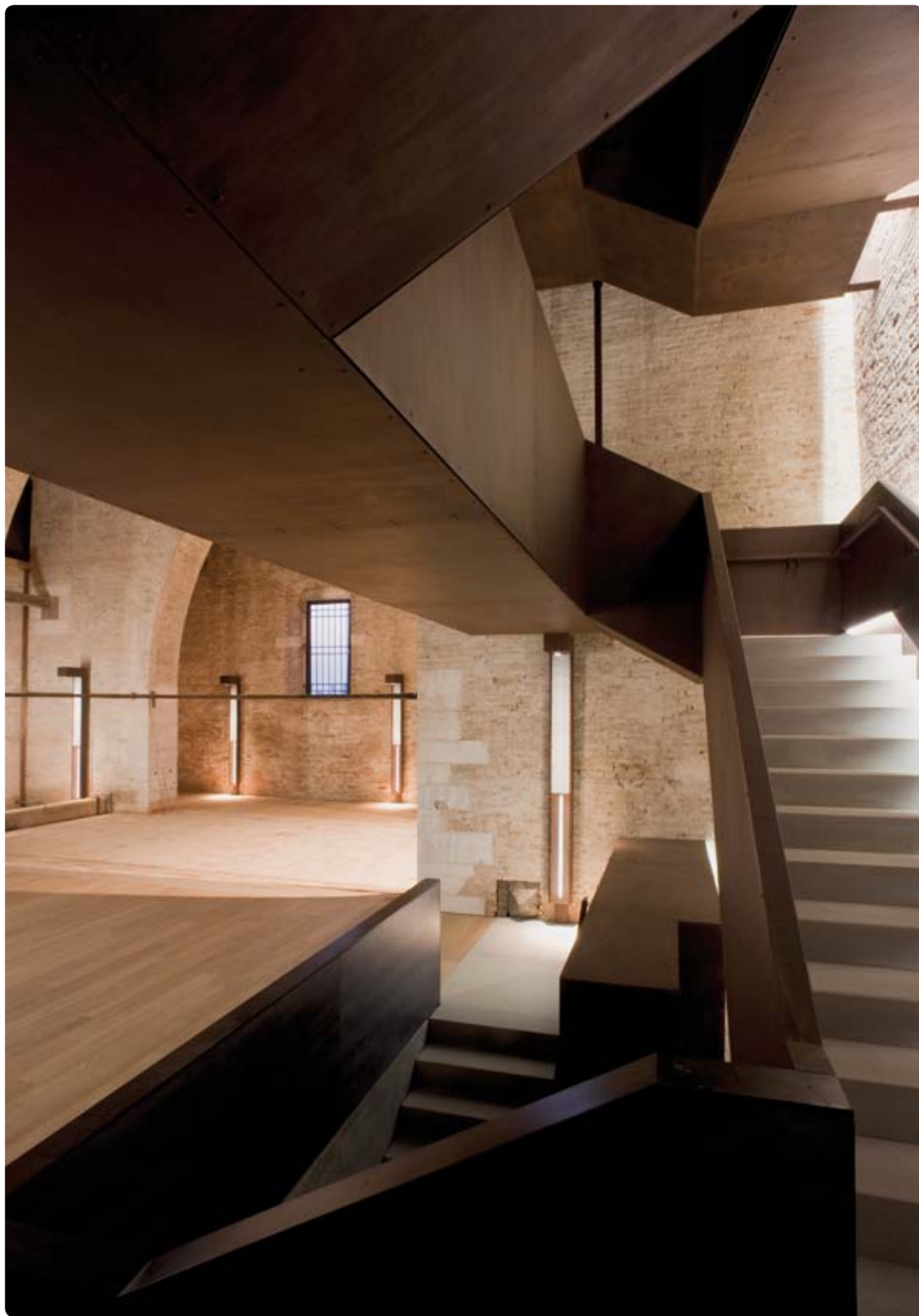
The new staircase is a self-confident intervention made of rough materials like iron and concrete.
