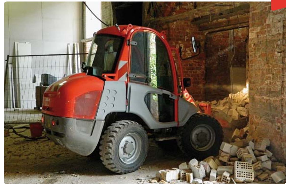
The beginning of the construction works
