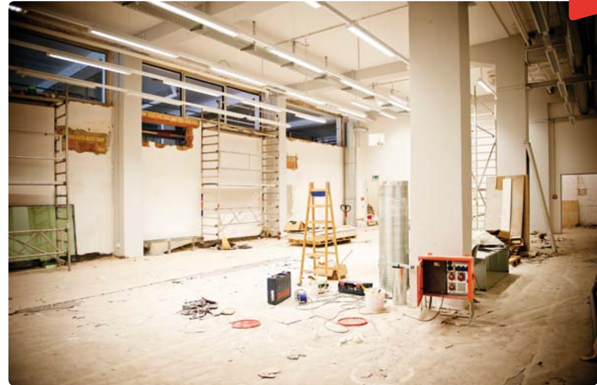
Werkstatt 141 during the construction work
